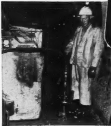
Gardner-Denver VP4 Sump Pump dewatering a tunnel under construction.
